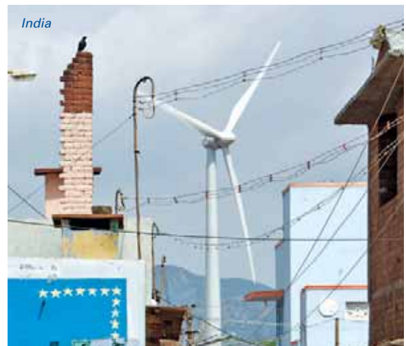
As of today, ReGen Powertech has erected more than 7.200 turbines – all of them featuring VENSYS technology.
